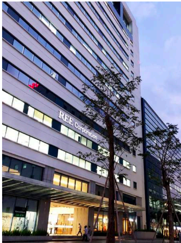
Image: e.town 5 building
